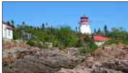
Otter Island Lighthouse, keepers' house, and the generator building
