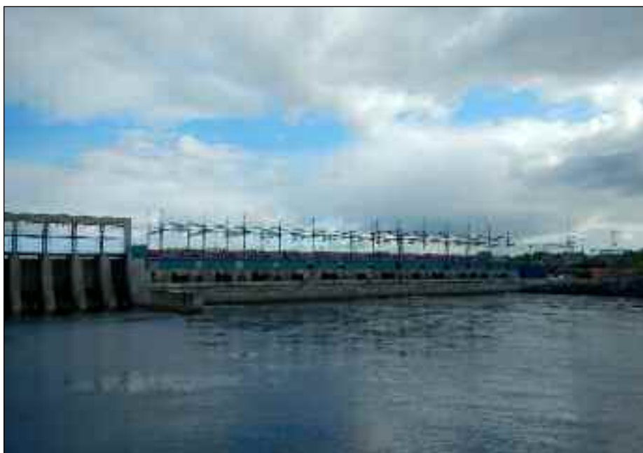
Dam and Powerhouse at Quebec Hydro's LG 1 facility
