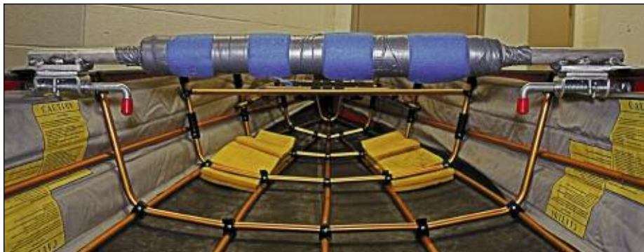
The new yoke installed
