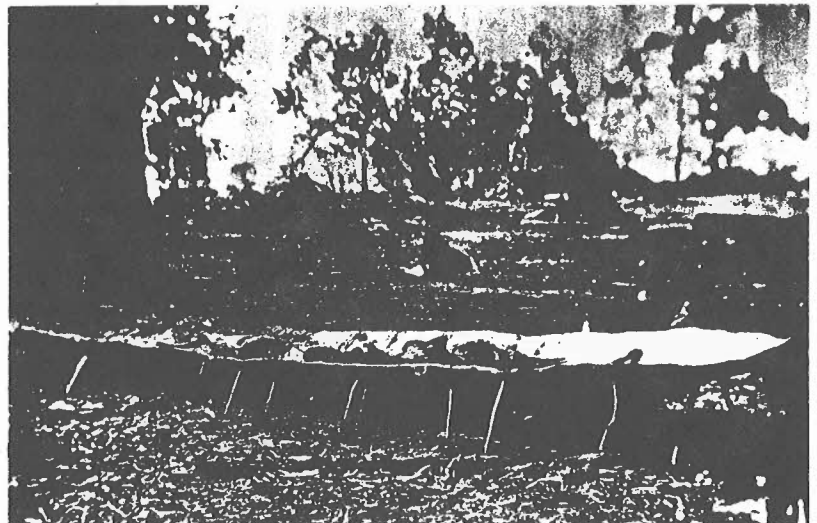
A bark canoe under construction at the Murray River in 1862. The bark sheet, propped up at the edges and with stones and logs to weigh it in the middle, was heated by fire underneath and inside. The heated sap made the canoe soft and pliable until it dried in the shape required
